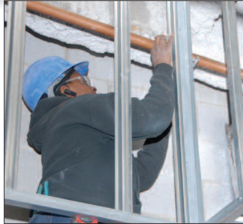
Plumber Frances Shaw runs water main lines
