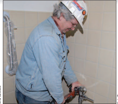
Plumber Doug Bryson tightens the flush valve
