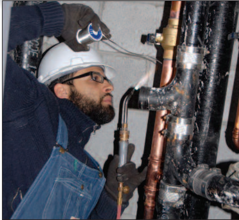
Plumber Joel Reyes operates a solder torch on ball valves
