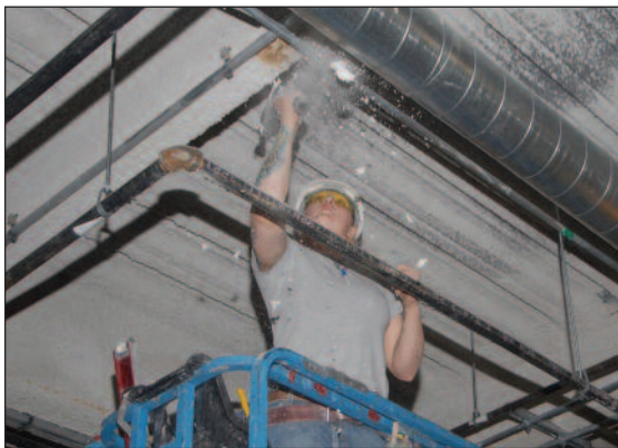
Rachel Morris Soffit installs courtroom ceilings
