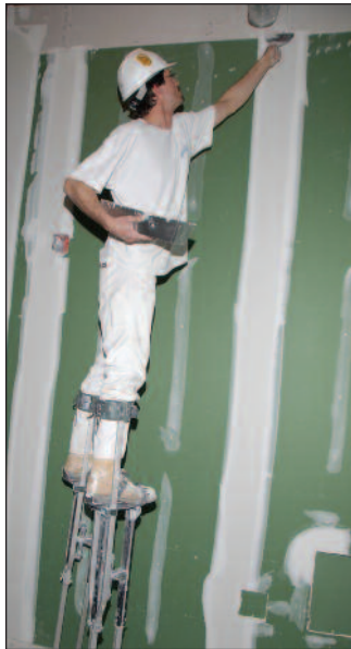
Rob Mauer on stilts taping drywall
