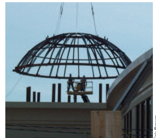
Dome steel support is lowered on base.
