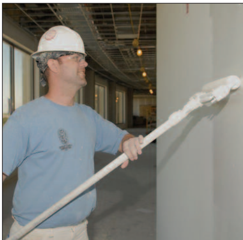
Kevin Fallon, painter, applies paint primer with an 18 inch roller
