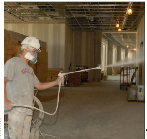
Painter Will Popowski sprays the wall with airless brush
