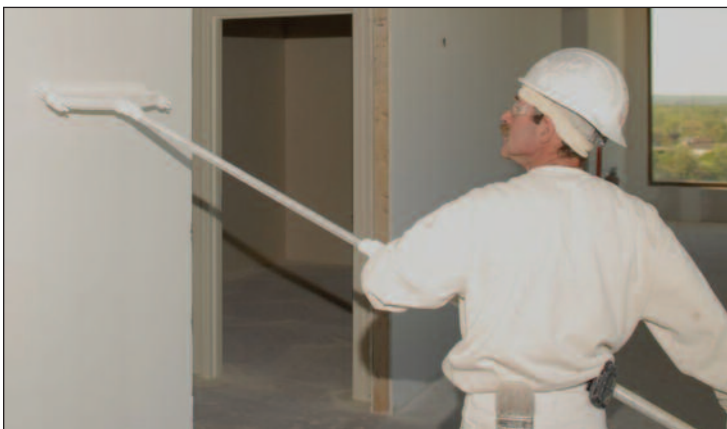
Painter Dennis Wielgosiek applies primer for litex, a specialty finish, on all public corridors
