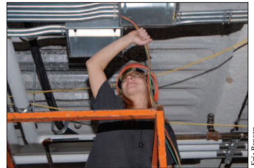
Erica Ferguson, electrician, performs lighting wire pulling
