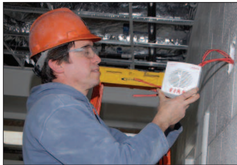
Pedro Ortiz installs fire alarm devices
