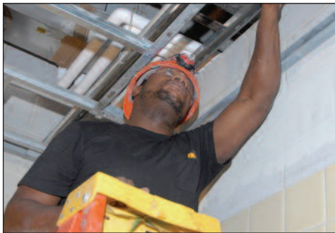
Electrician James Sawyer places light fixture supports
