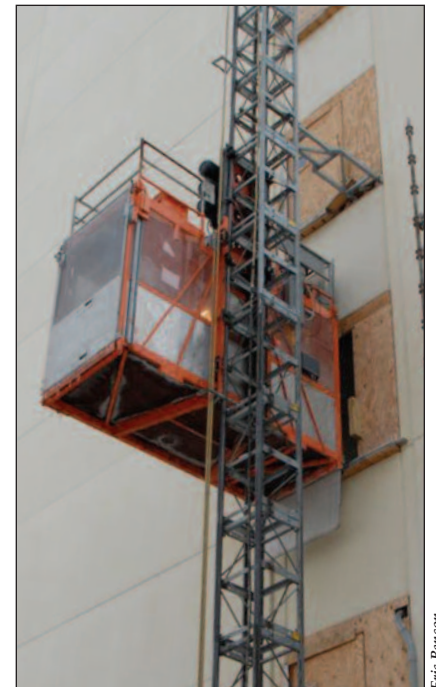
The buck hoist travels up and down the building
