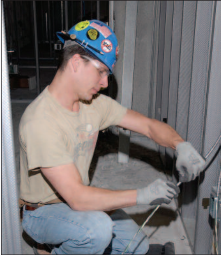
Electrician Gary Gubanich runs cable through metal studs for office receptacles
