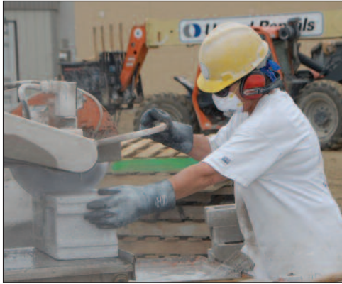
Dawn Precht, brick mason, operates masonry wet saw
