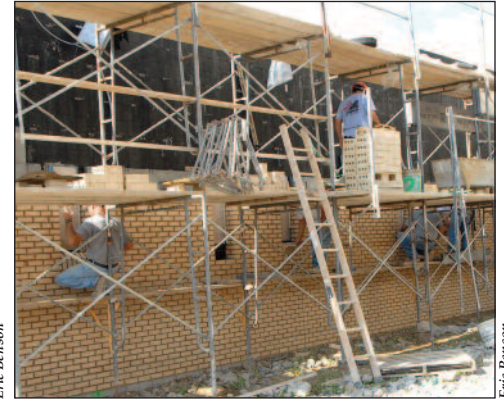
Several masons lay brick seals and veneer on outer JJC wall
