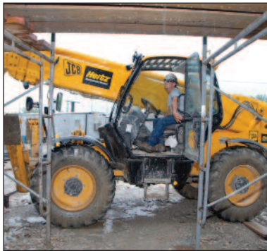
General Labor Foreman Tim Montalvo moves heavy loads with the lull
