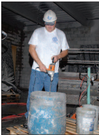
Ed Miller mixes and tends plaster for fireproofing
