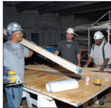
Laborers Larry Caver, Dave Martin and Allen Jones cut wood for swinging door with circular saw
